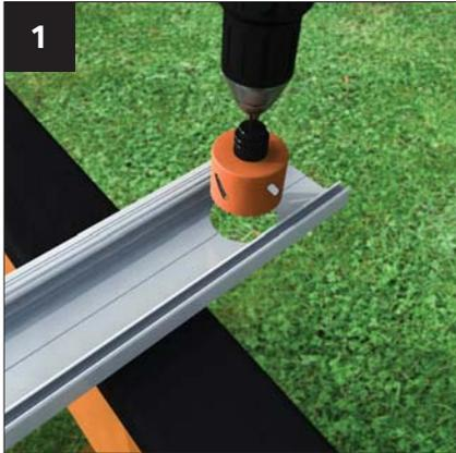
Decide the position of the gutter outlet by lining the extrusion 'v' groove up with the centre of the hole for the down pipe. Using a 73mm dia hole saw, cut the hole for the down pipe in the lower section.
