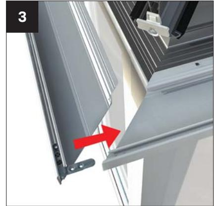
Fit the cleats (CRN001) to the desired side using the fixings provided (CRN006) as shown and assemble the remaining lower sections
